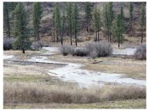
After a spectacularly snowy winter the other shoe fell with extremely high runoffs this spring. The wetland mitigation project on the Meyers Place along the South Fork of the Palouse River performed as designed. The river breached the lowered river banks and filled the holding ponds
